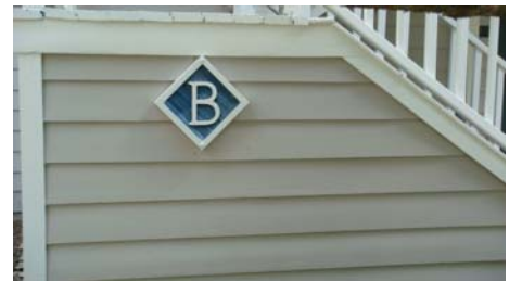
BRANDON RIDGE CONDOMINIUMS - After
